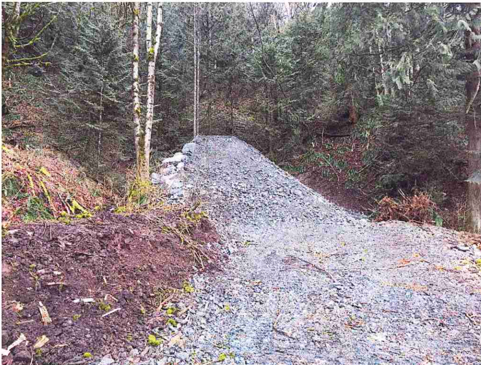
Photograph 14. – Protective berm viewed to the west.
