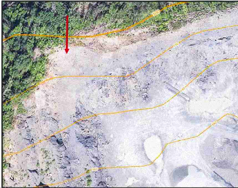
Figure 4: The 2016 imagery showing approximate location of the initiation zone marked with a red arrow. The new turn around area extends to the north within the initiation zone.
