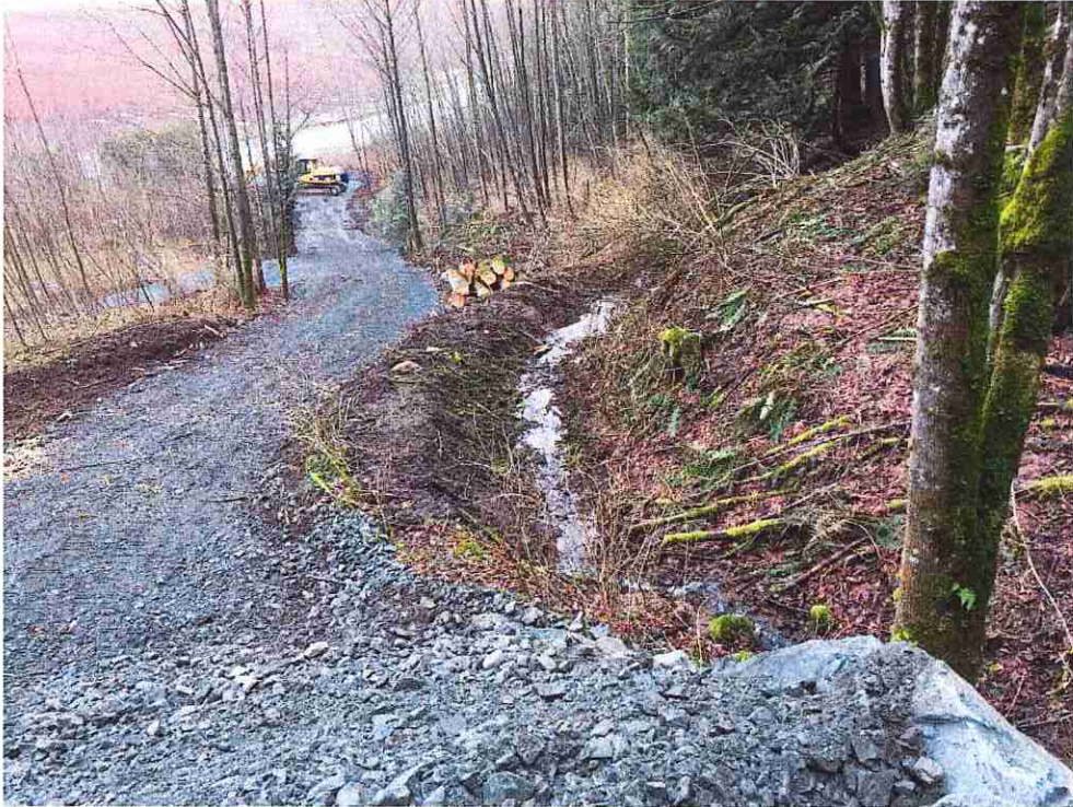
Photograph 16. – Ditch east of protective berm.
