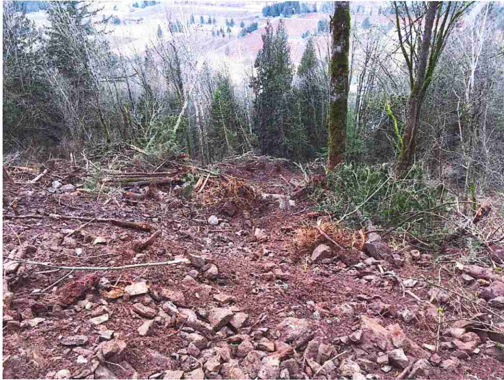
Photograph 9. – Loose cobbles and boulders downslope of Vedder FSR.
