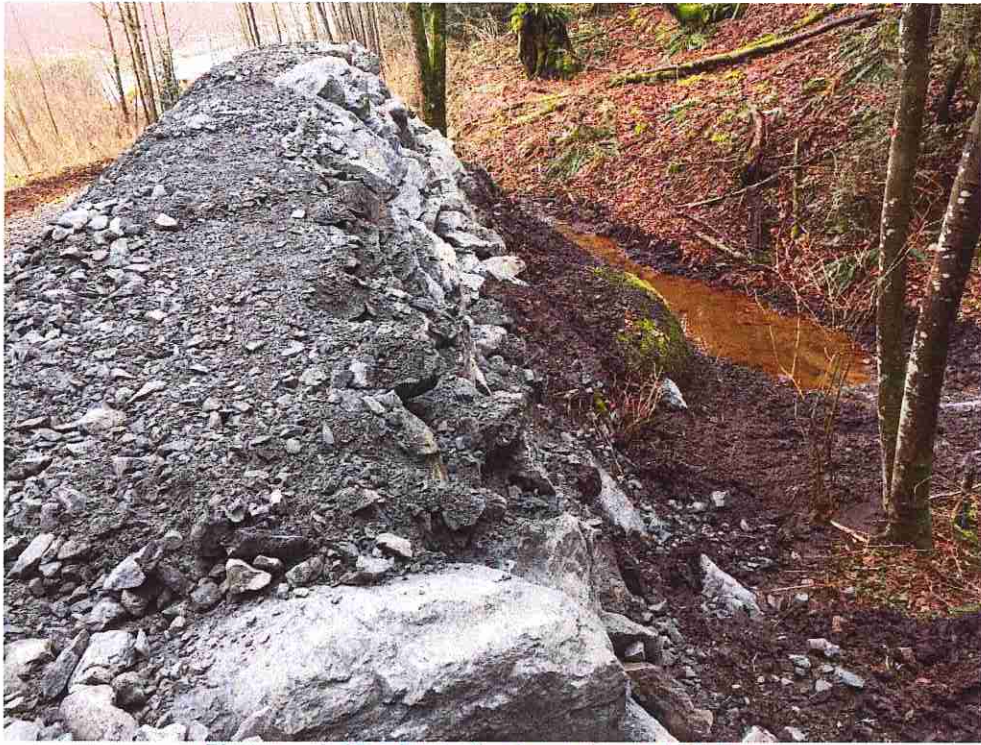
Photograph 15. – Protective berm viewed to the east.
