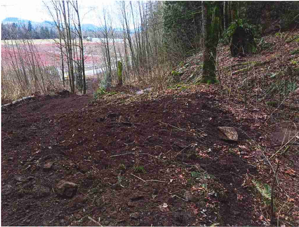
Photograph 13. – Existing berm built prior to debris flow with diversion ditch conveying flows towards 44100 VMR to east.
